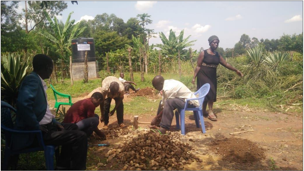
5.0 Community preparing local ballast for slab casting at Imani Bora village
