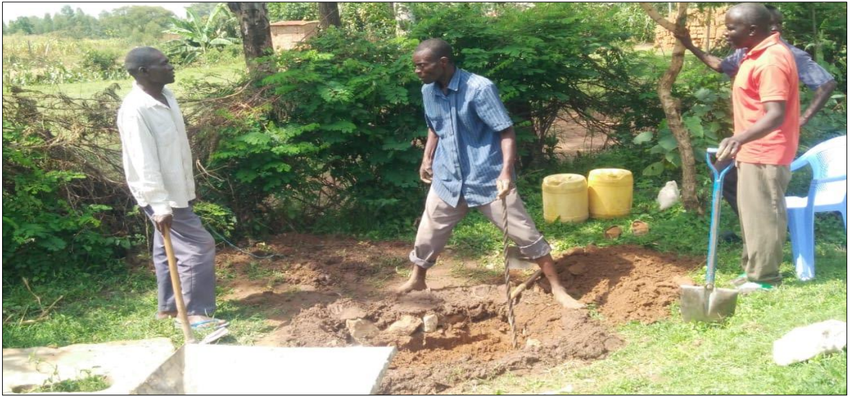
7.0 Preparing latrine site for mounting of slab for latrine construction
