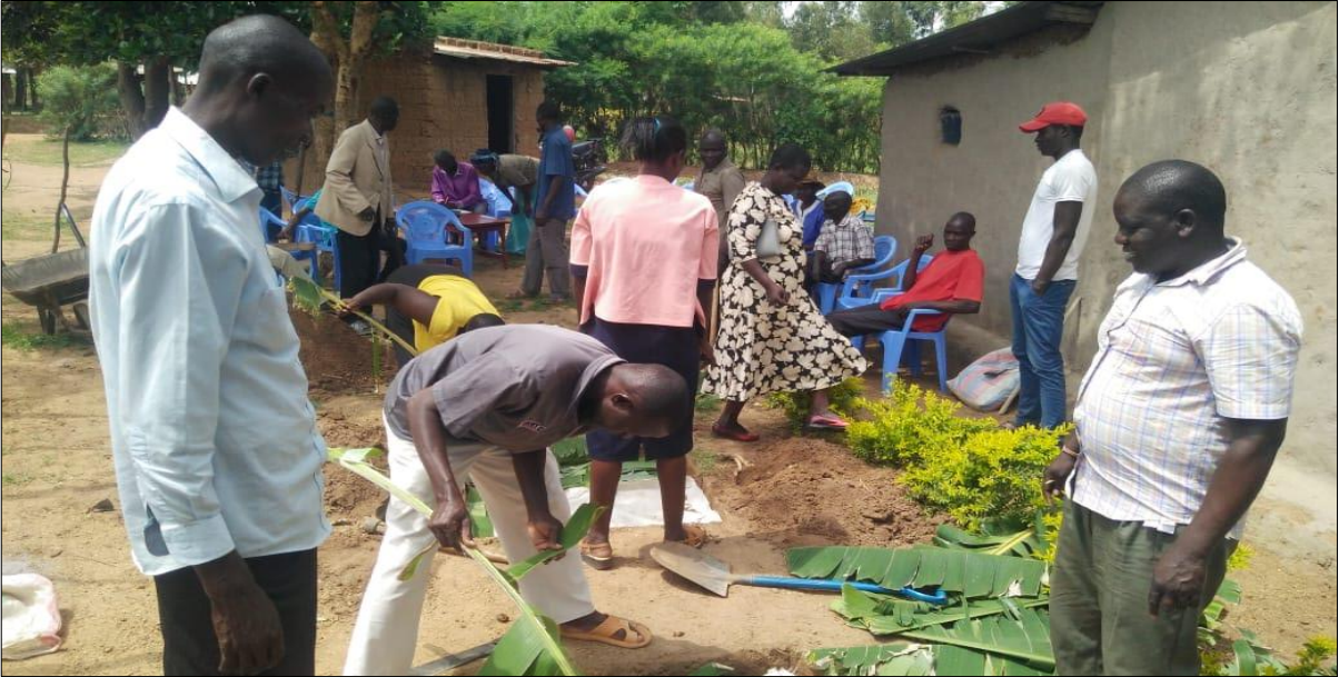
9.0 Community members casting SAN PLAT slabs for latrine construction
