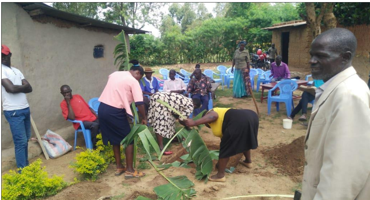
4.0 Community members preparing site for slab casting at Imani Bora Village
