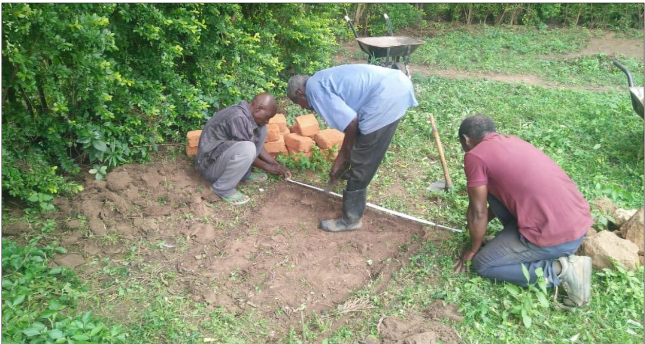
6.0 Preparing site for slab casting at Bititi Youth group village
