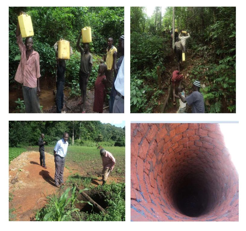
In the picture above is the beginning of digging the bore hole at Bisaju. But this hole could not be completed because of the hard rock found at 5 feet after top soil. This forced to shift to about 1 km from here.
