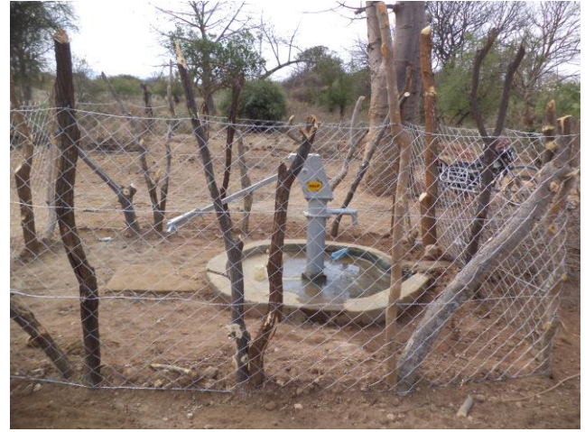
Nguni Borehole after Rehabilitation
