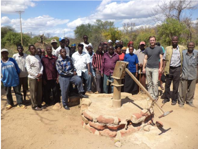
Nguni Borehole before Rehabilitation
