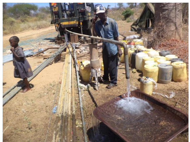
Complete borehole rehabilitation and six hours of recharge testing at Nguni
