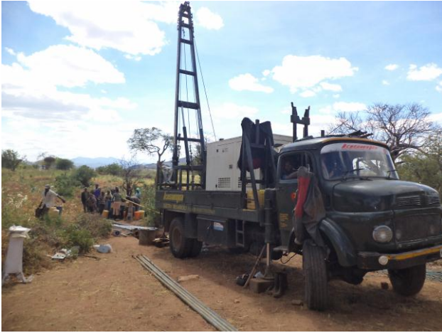
Complete borehole Rehabilitation and Six hours recharge testing at Kamuthale
