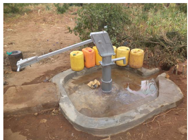
Kamuthale Borehole After Rehabilitation
