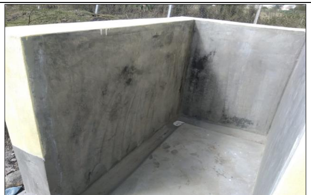
6. Construction of Urinals for the boys
