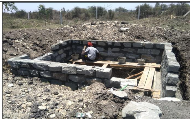
3. Construction of the foundation walls & ring beam for the boys' latrines
