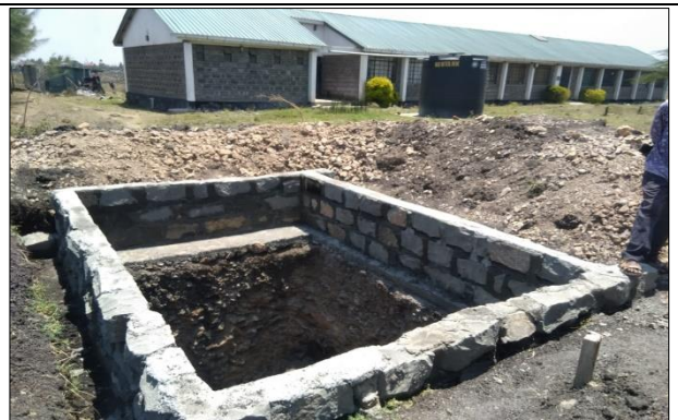
4. Girls latrines ready for slab construction
