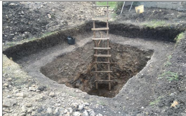
1. Excavation of the pit latrines
