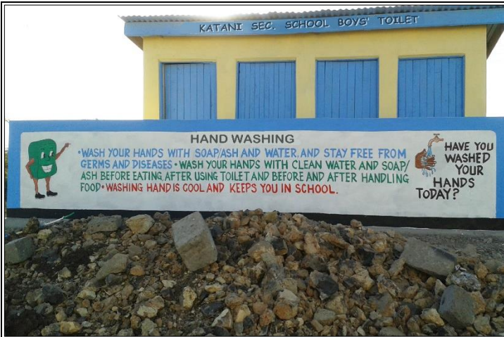
7. FRONT VIEW OF THE BOYS VIP LATRINES WITH HYGIENE & SANITATION MESSAGES
