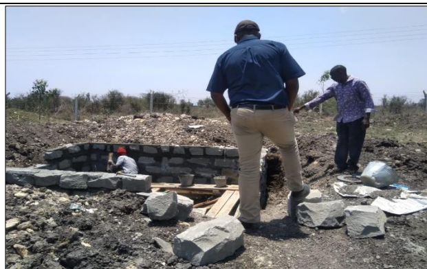
5. KUMEA Staff inspecting construction works
