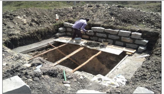
2. Construction of the foundation walls & ring beams for the Girls latrines
