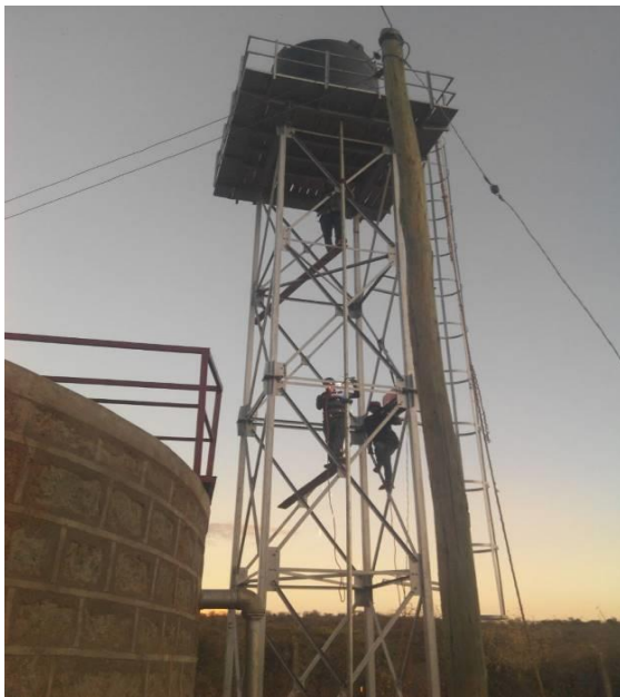
Elevated backwash tank installation
