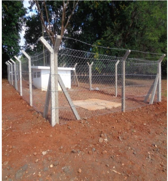
Fencing of the pump house to keep away intruders
