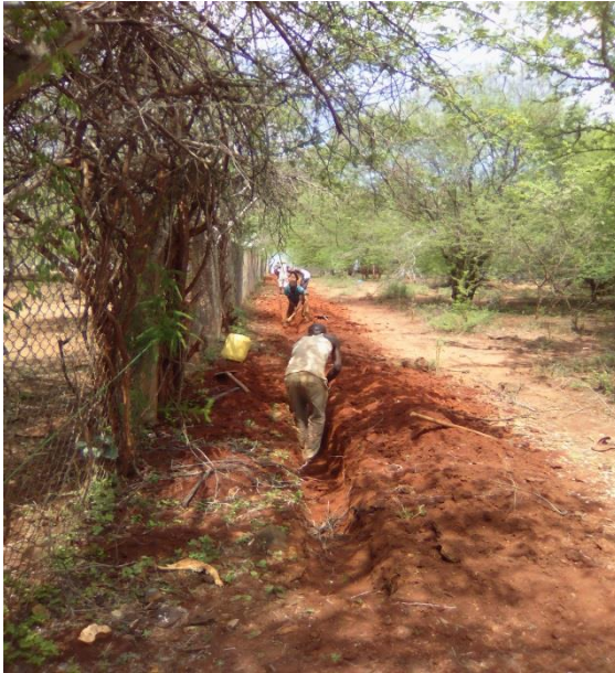
Pipe trench excavation close to the dam
