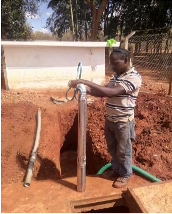
Installation of the submersible pump at the sump
