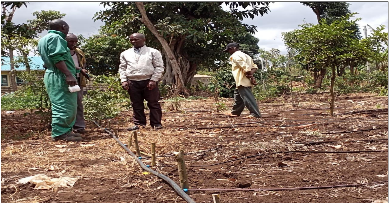
8.0 Installation of drip irrigation system at Thaicu mixed Secondary school
