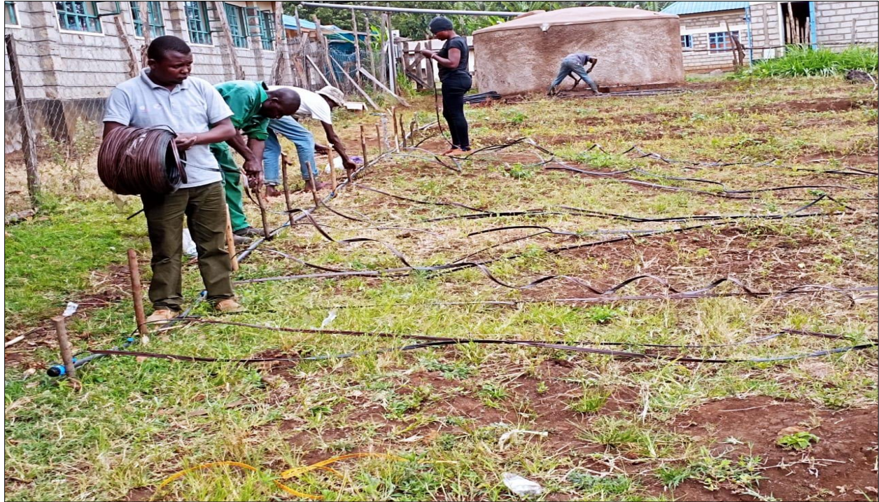
9.0 Drip irrigation system installation at Karumaru Secondary school
