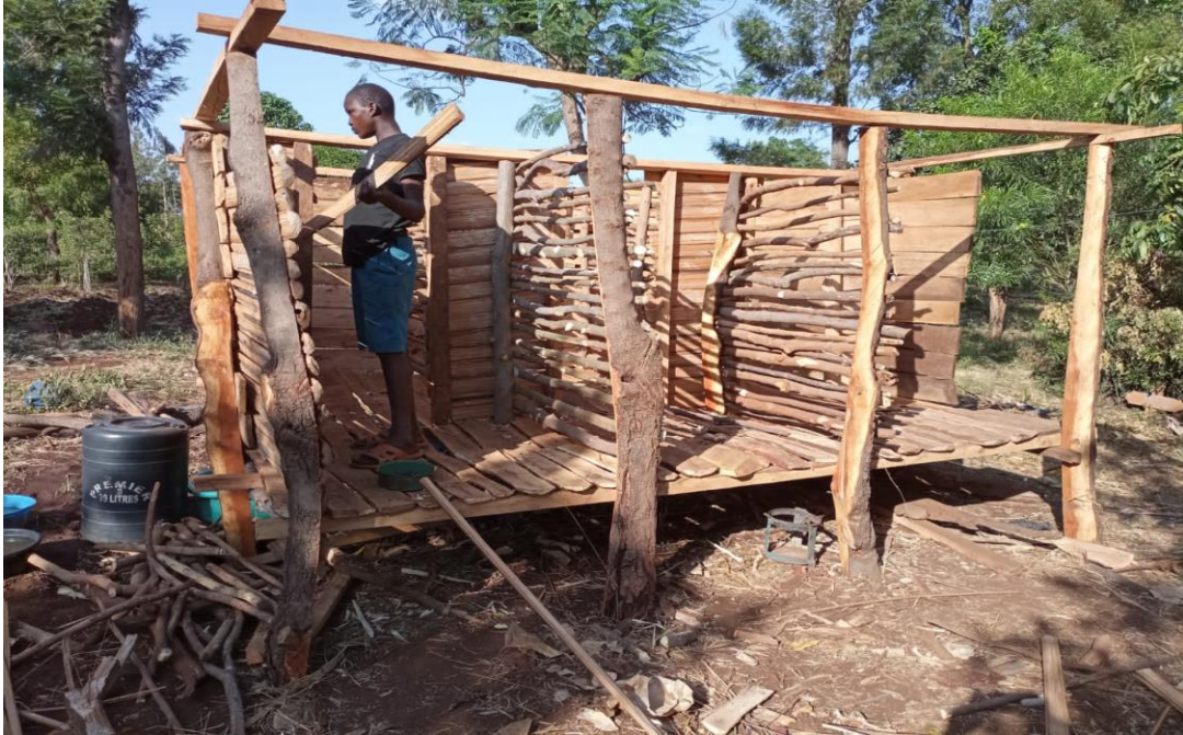
10. Group members of Wendo Mweiga women constructing their animal pens/shades in preparation of the Dairy goats to be received from the project
