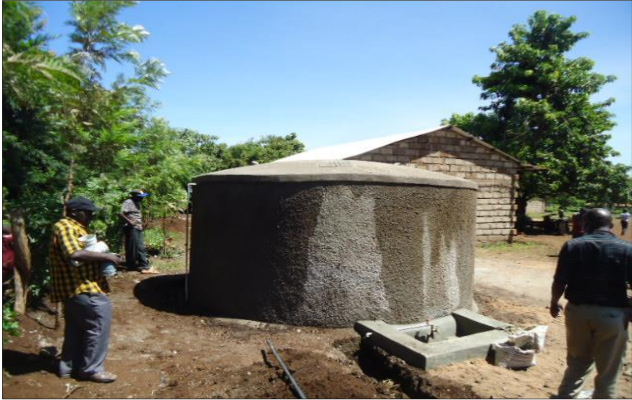
5.0 Completed 30,000litres Ferro-cement water tank at Nkiri Primary school to facilitate horticulture &agroforestry in the school
