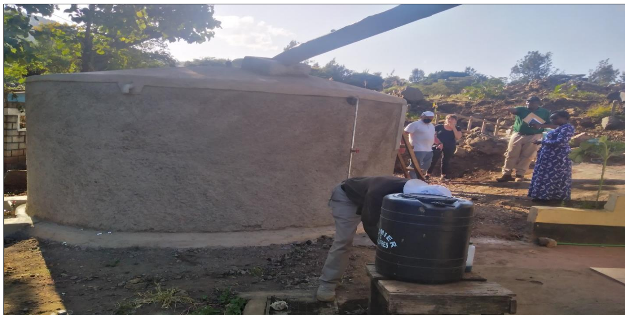
7.0 Completed 30,000litres Ferro-cement water tank at Nthare Secondary school to facilitate horticulture &agroforestry in the school
