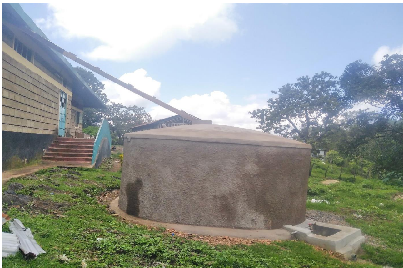
7.0 Completed 30,000litres Ferro-cement water tank at Nthare Secondary school to facilitate horticulture &agroforestry in the school
