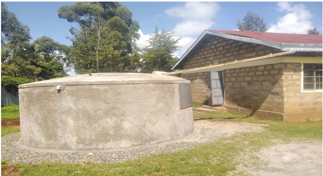
5.0 Completed 30,000litres Ferro-cement water tank at Nkiri Primary school to facilitate horticulture &agroforestry in the school
