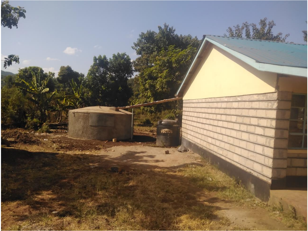
9.0 Completed 30,000litres Ferro-cement water tank at Thaicu Secondary school to facilitate horticulture &agroforestry in the school
