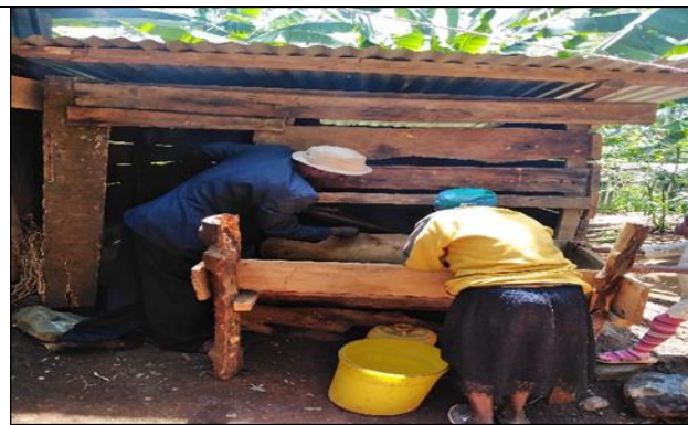
3. Inspection of the completed animal stable/pen for Kamanu Women group member
