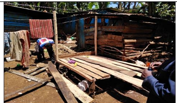
5. Construction of the animal stable/pen for Wendo Mwega women group member
