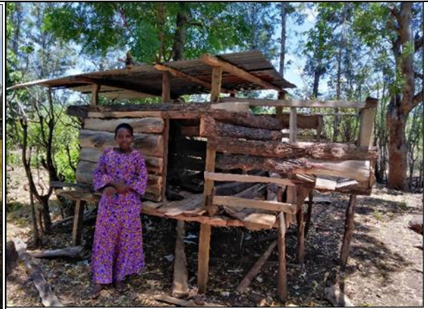
2. Wendo Mwega women group member completed construction of the animal stable/pen
