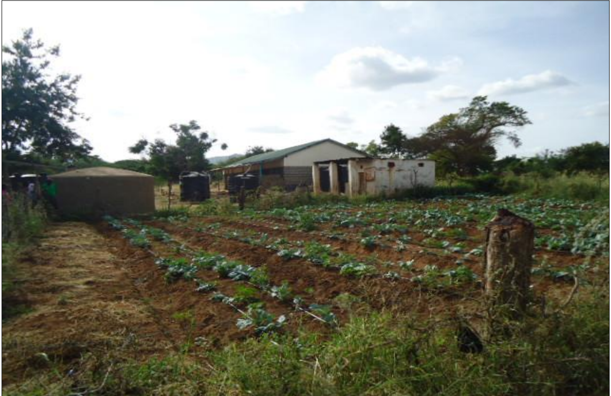
4.0 Ferro-cement Water & Drip irrigation system providing water for the school agriculture demonstration farm
