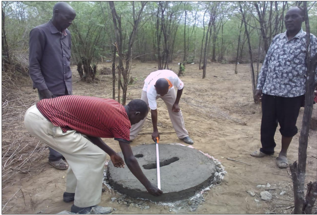
6. Preparing circular SANPLAT slabs & taking measurements for household latrine construction
