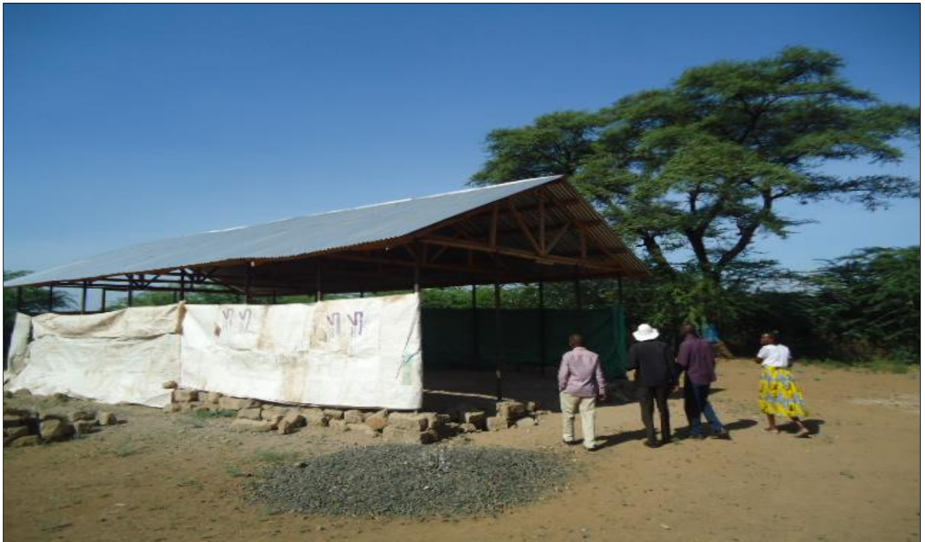
5. Eldume ECD School after reconstruction
