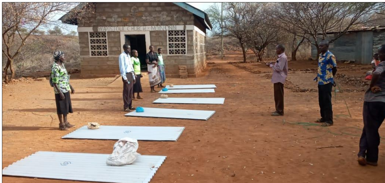
1. Distribution of roofing materials &nails to vulnerable households displaced by floods in Loruk and Monoini villages
