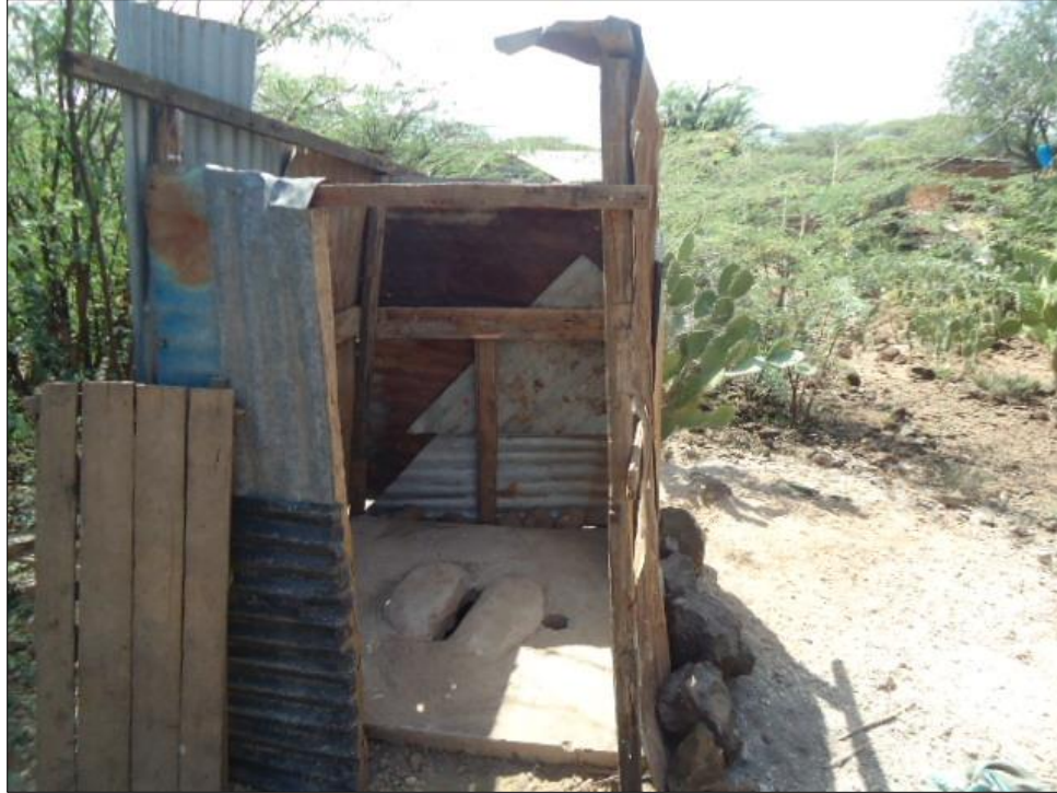
13. Temporary structure household latrine with SANPLAT Slabs in use in Ngenyin village
