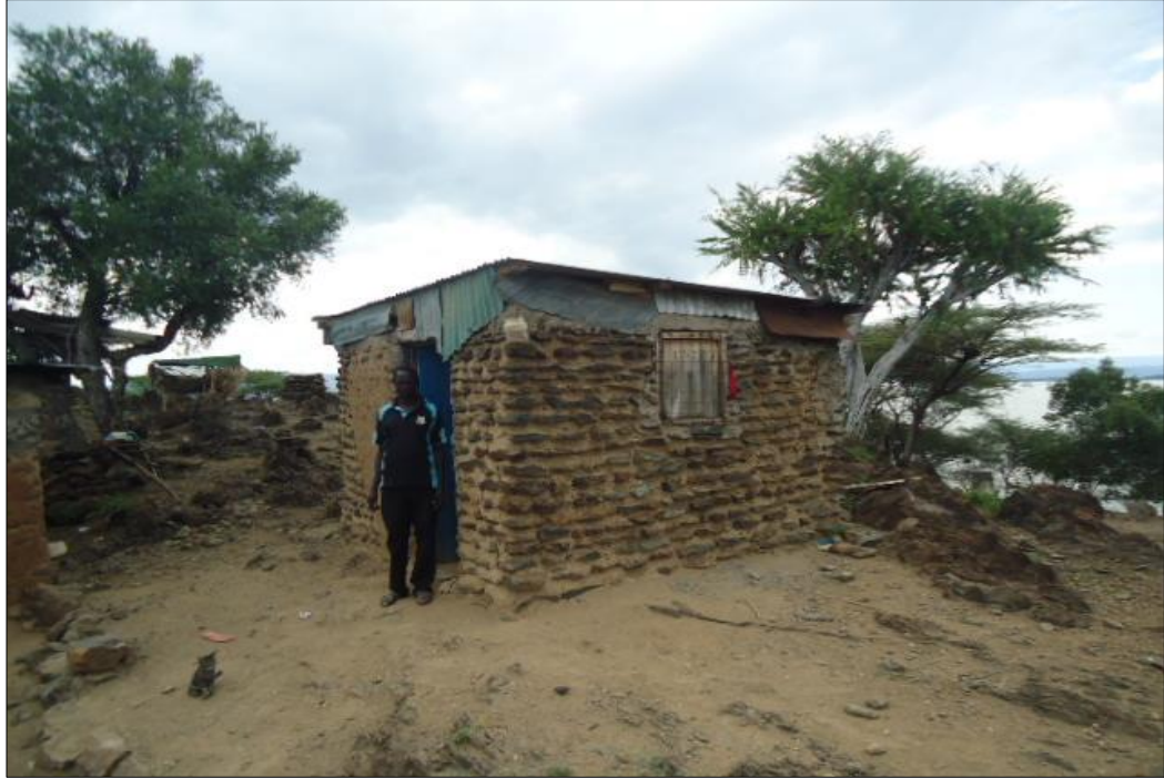
7. Vulnerable household Pius Chelimo accessing a reconstructed house supported by the project in Ngenyin village
