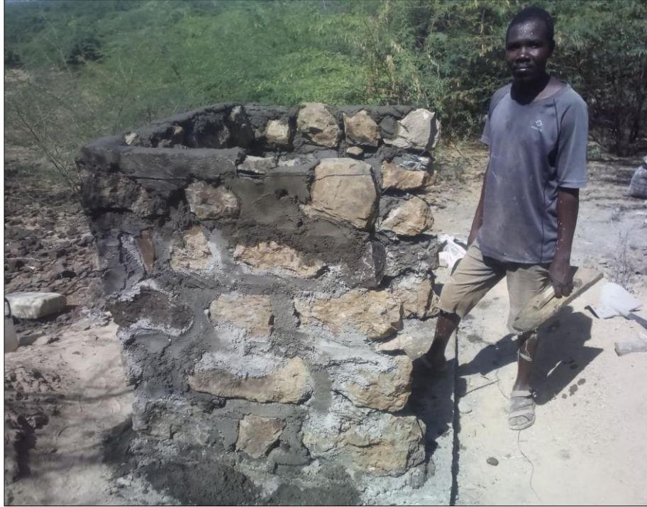
8 Household latrine construction for vulnerable displaced household in Ngenyim village
