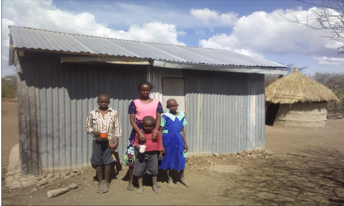
5. A vulnerable household & family affected the floods supported to construct a house in Salabani village
