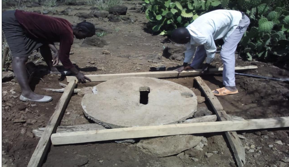
3. Preparing SANPLAT slabs for construction of improved latrines
