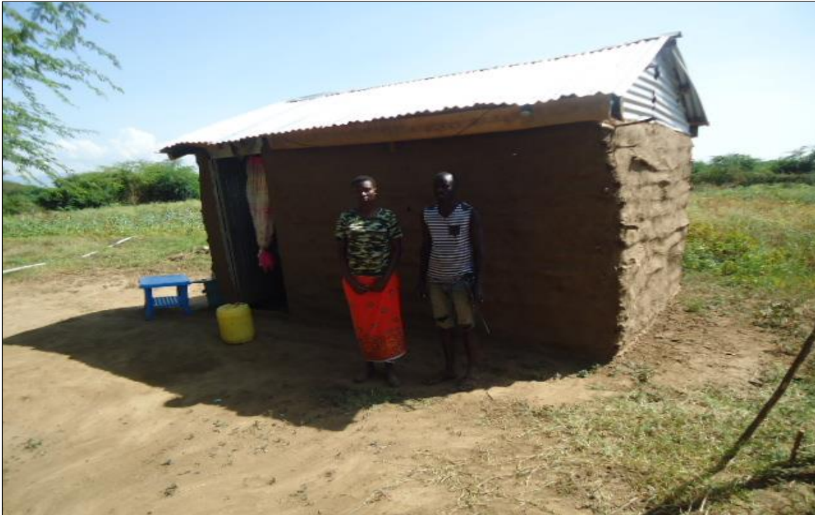
11. A vulnerable family Ms. Josephat Lenaso who relocated due to floods have been supported by the project to construct a house in Eldume village
