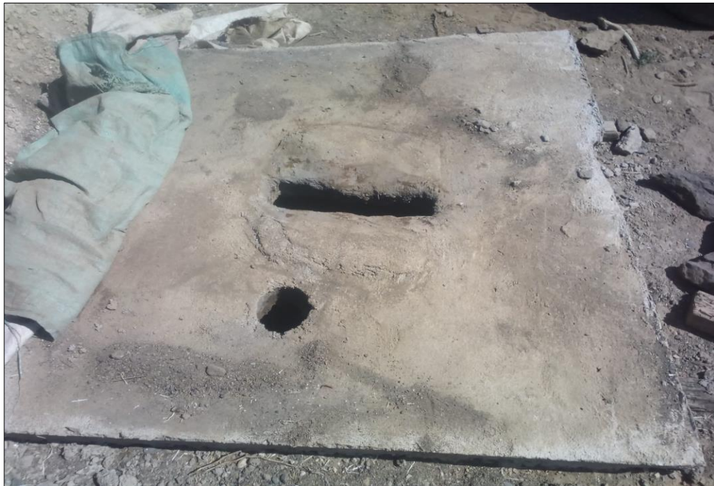
7. Rectangular SANPLAT latrine slab ready for household latrine construction
