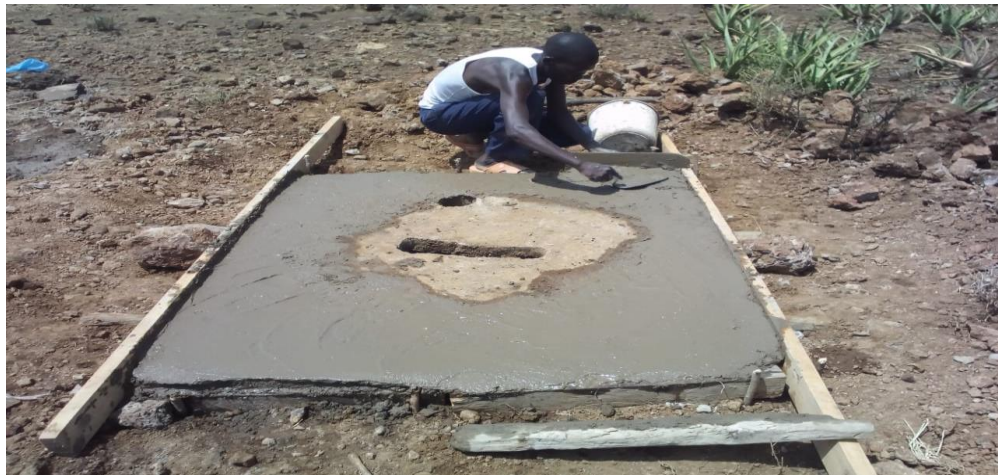
4. Construction of the Households latrines in Salabani village
