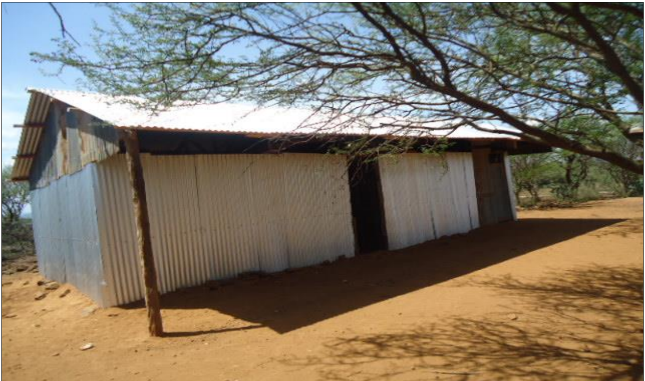
7. Monoinin Primary School ECD Center classroom reconstructed after relocation due to floods
