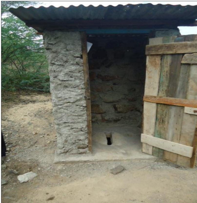
9. Completed latrine and in use in Ngenyim village for displaced vulnerable household
