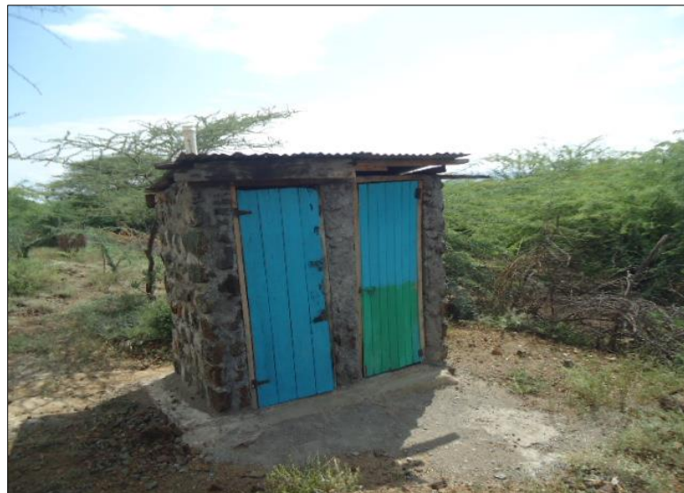
12. Completed household latrine for vulnerable displaced households in Moinini village
